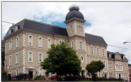
BIS Building, St. Patrick's Hall, St. John's, Newfoundland
